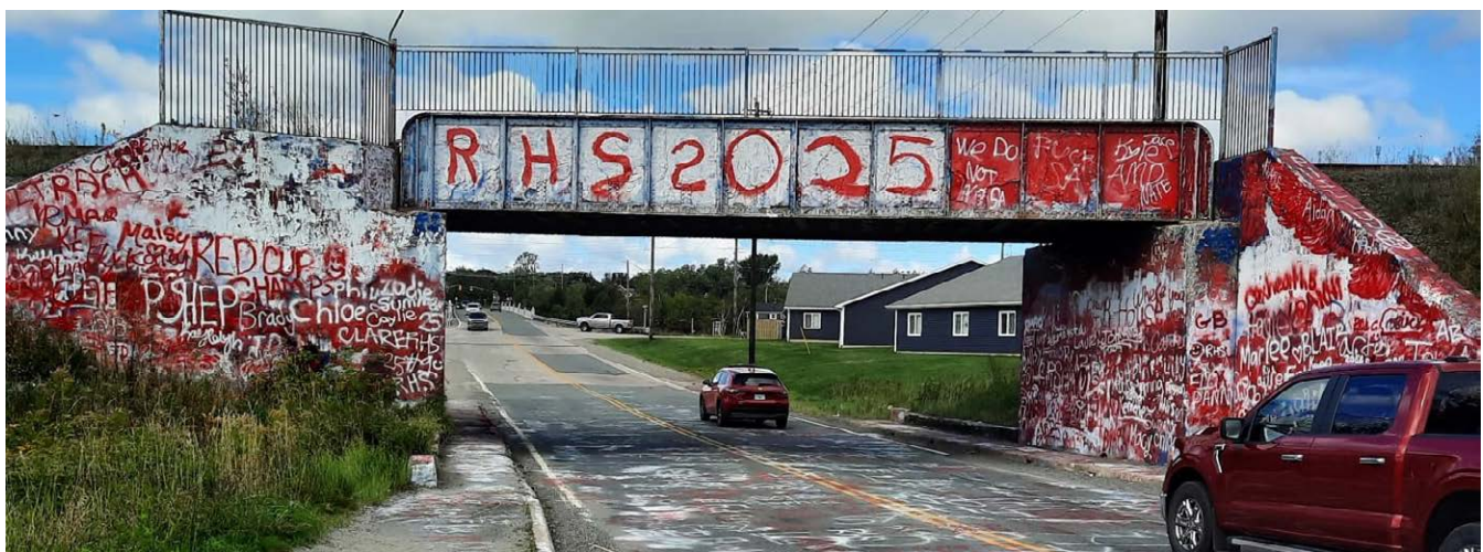
Photo 23 - Keltic Drive Underpass
