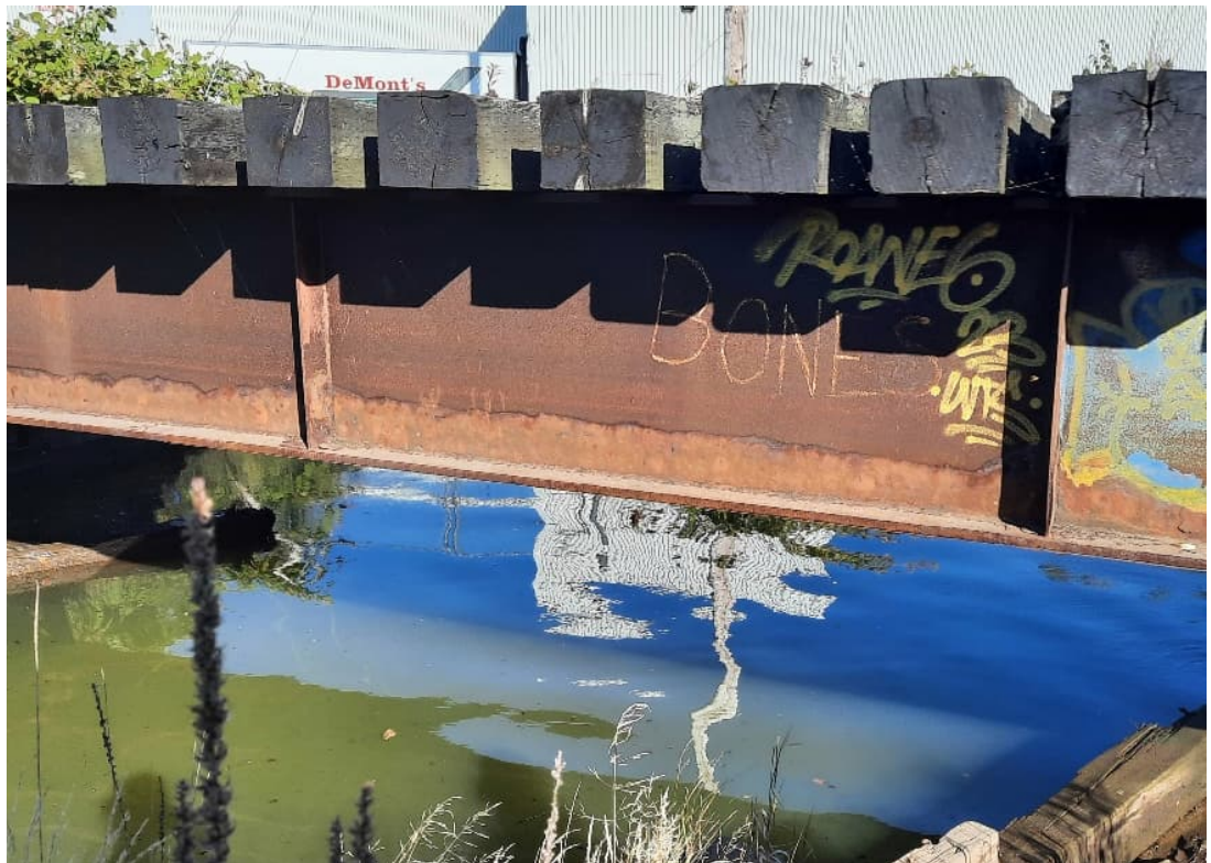
Photo 26 - Muggah Creek Bridge
