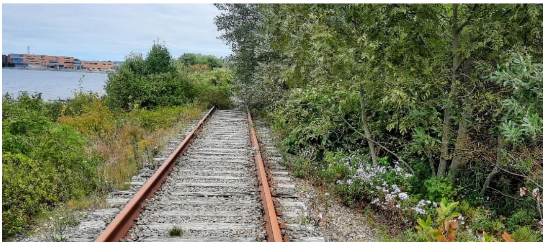
Photo 2 - Ballast and Surfacing
