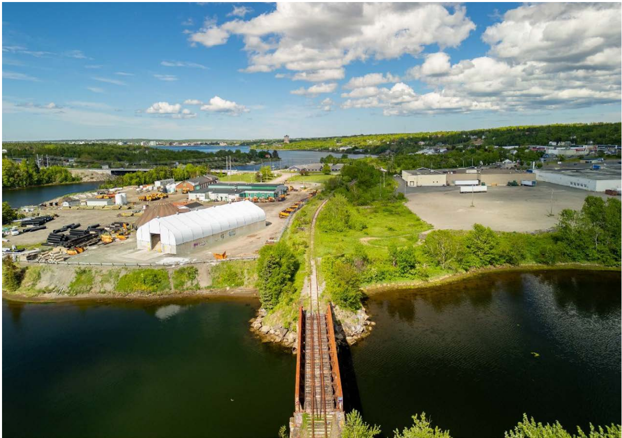
Figure 4: Overview of the Existing Tracks Crossing Sydney River
