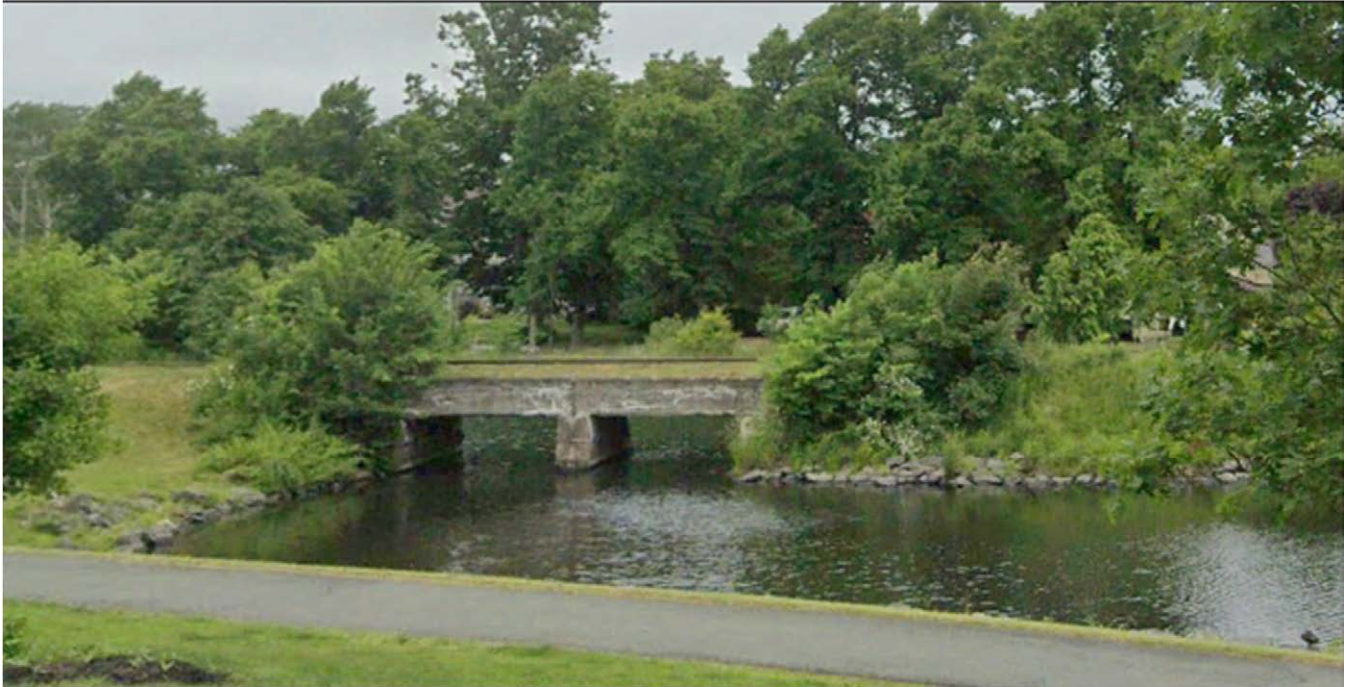
Photo 25 - Wentworth Park Bridge
