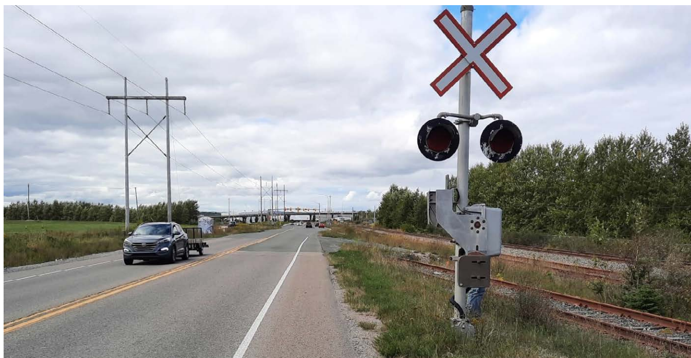
Photo 18 - Sydney Port Access Road
